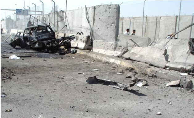
Fig. 7a: Damaged protective wall after VBIED attack
