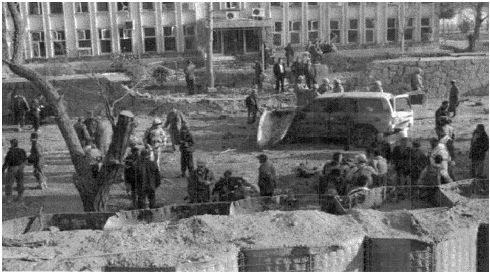
Fig. 7 Comparison of damages on rigid and loose protection structures (archive of the author)
